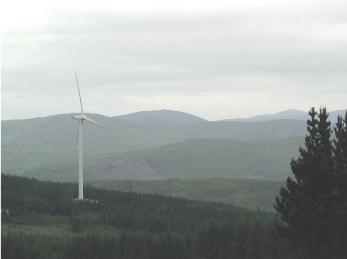
Photo of a Vestas V90 in Montaigne environment.
